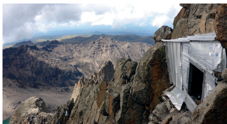
The Baillie bivy, used far less frequently following the construction of the Howell hut. ( Nicholas Hurndall Smith )
